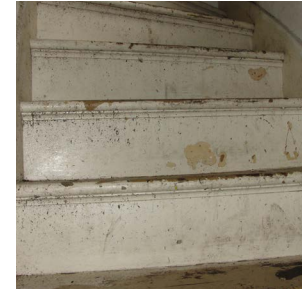
Before lead paint interim controls
