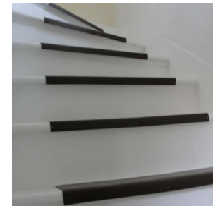
After lead paint interim controls
