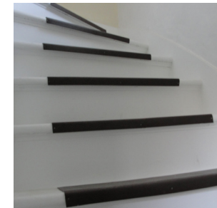
After lead paint interim controls
