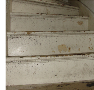
Before lead paint interim controls
