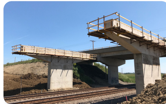
Construction of the new bridge over the Canadian Pacific Railway
